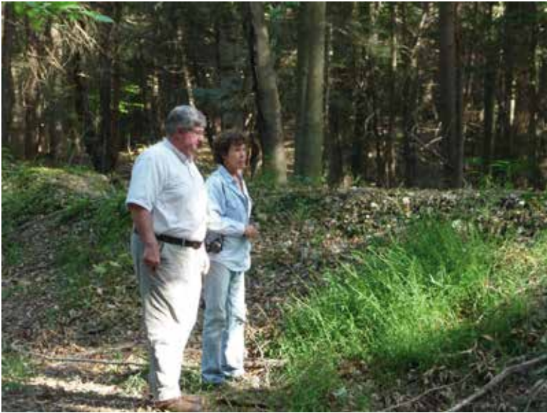
Jim Zeoli and Selectman Judy Wright Williams inspect the Berm protecting Surrey Drive.
